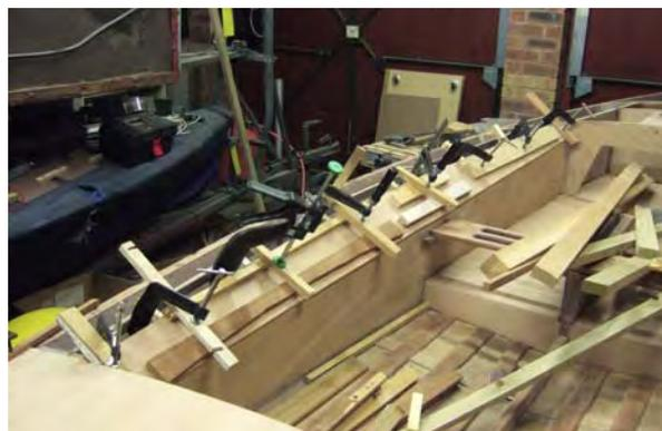
*Sloping side decks glued and clamped (Photo: Matt Whitfield)*
